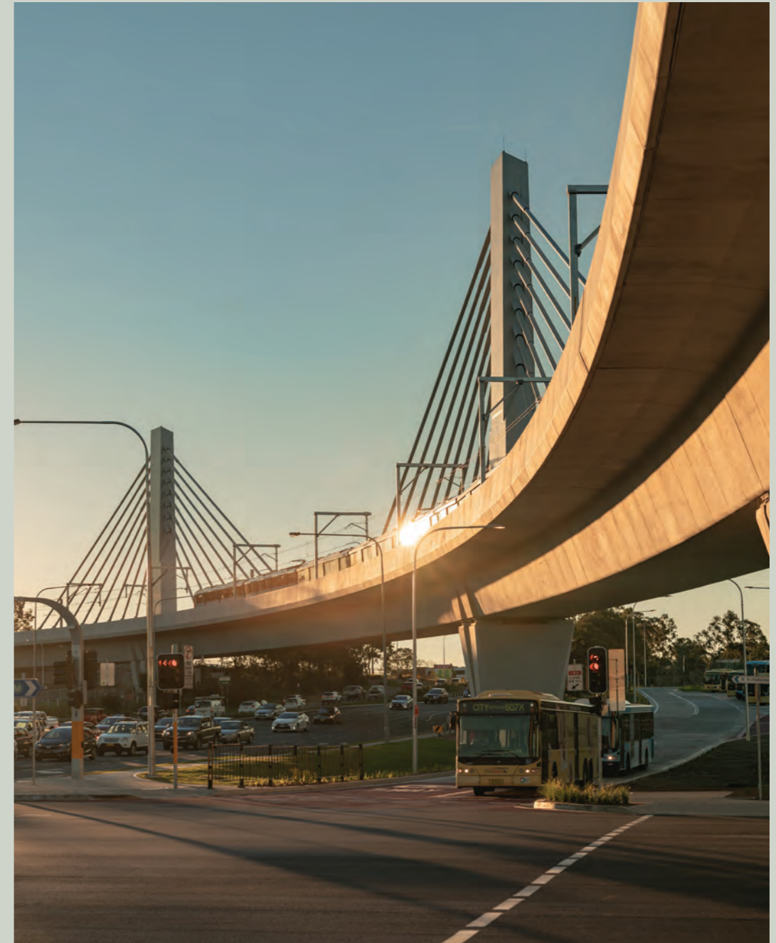
ROUSE HILL BRIDGE
